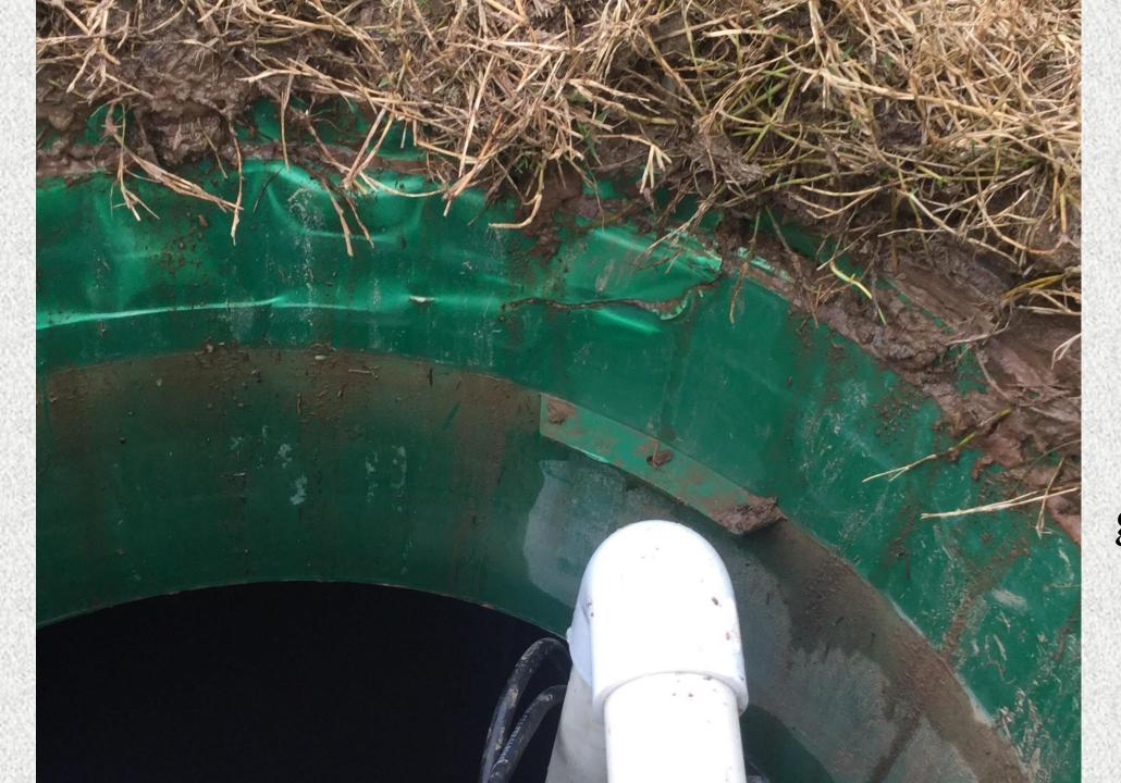
Cracked riser  $\rightarrow$ leaky tank  $\rightarrow$ groundwater in tank
